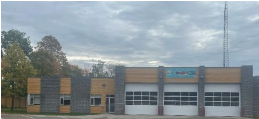
Figure 8. Exterior of Station 1 – Brownsville.
