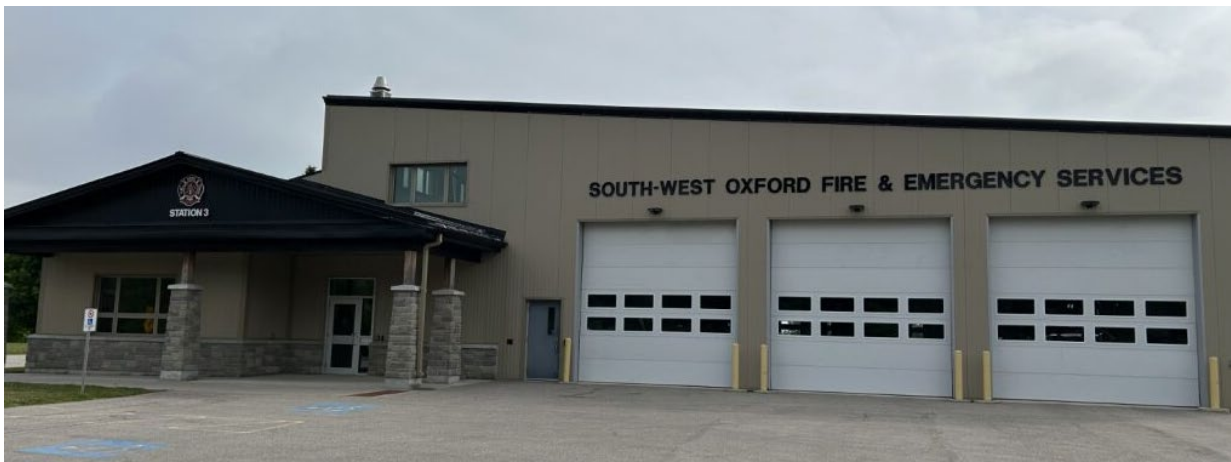
Figure 10. Exterior of Station 3 – Beachville.
